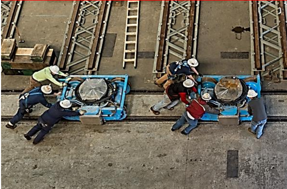
Manually push transfer cars (380+ lb init. force, 150+ lb of sust. force)
